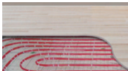
Floor Heating Coil
